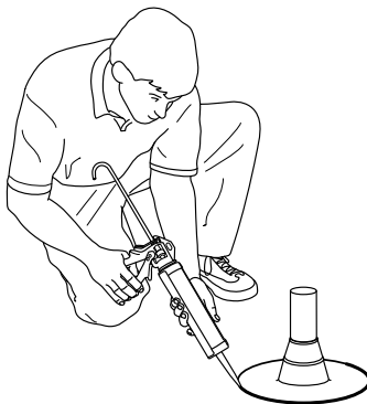
After cleaning around the boot flange, caulk the edge.
